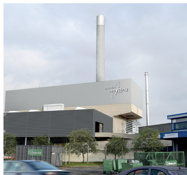
Eastcroft EfW plant in Nottingham (United Kingdom)
